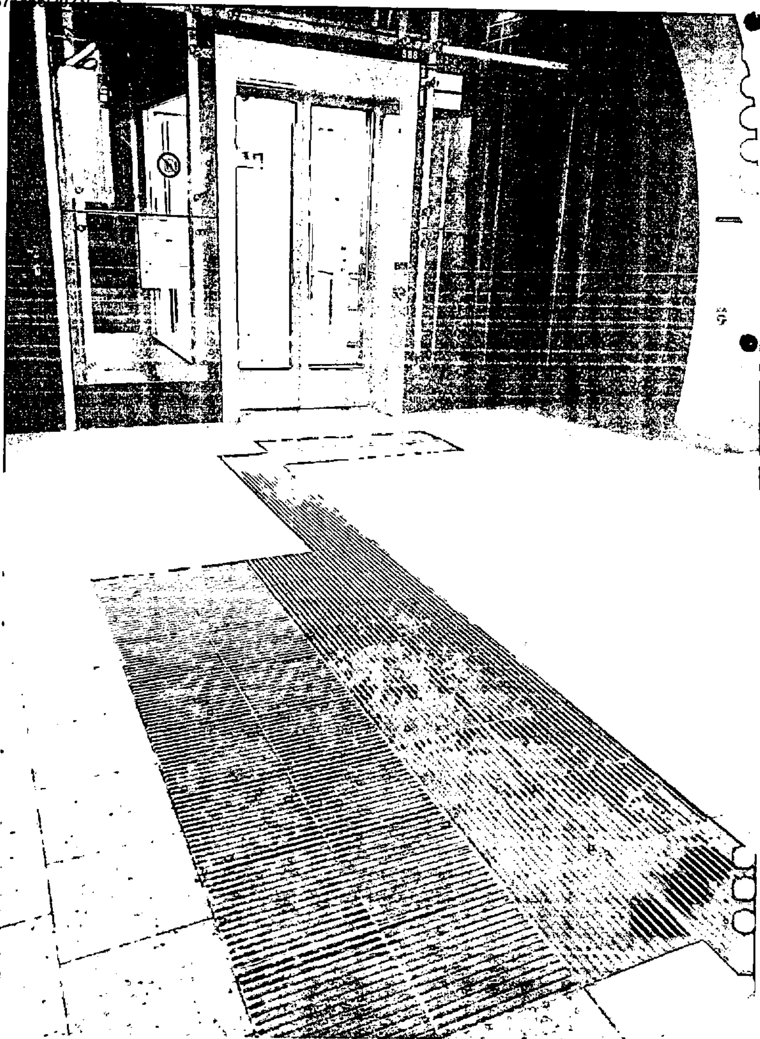
Image 4.9 Tactile pavers layout towards the lifts access Photo Credits: Dr. Gaurav Raheja
