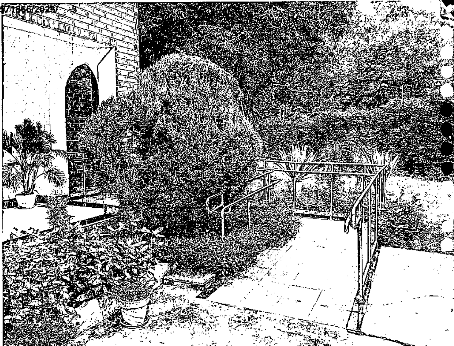
Image 7.6 Retrofitted ramp as an accessible entrance of a guest house Photo Credits: Dr. Gaurav Raheja
