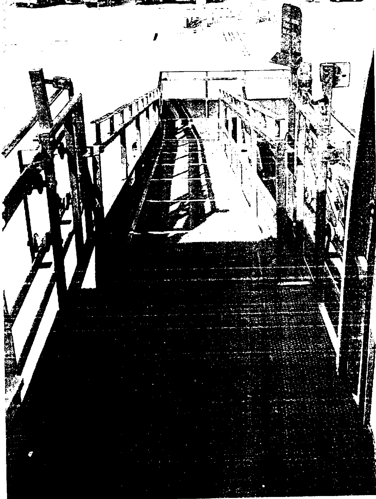
Image 6.30 Accessible ramps for aircraft boarding Photo Credits: Saraya Shetty
